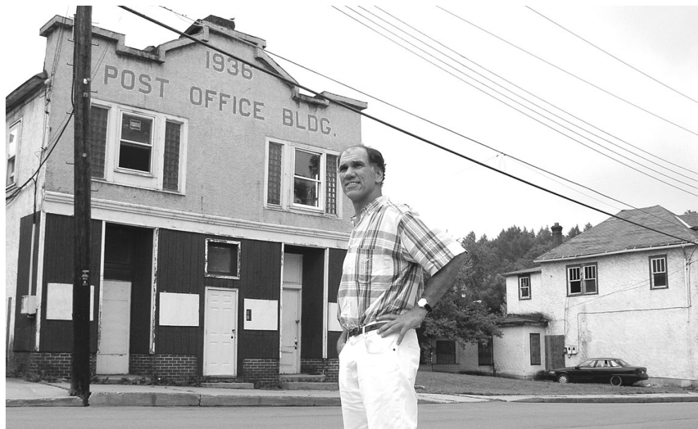
MOUNTAINDALE'S DOWNTOWN has its own marketing manager. Bob Shrem, who lives on the hamlet's Main Street, is outside a dilapidated shell of a building which is slated to be turned into nine SoHo (small office/home office) apartments. BARBARA GREFF PHOTO
