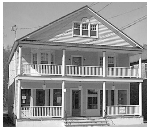
NUMBER 51 Main Street in Mountandale (shown before and after) has been called one of the best downtown renovations in Sullivan County. PROVIDED PHOTOS
