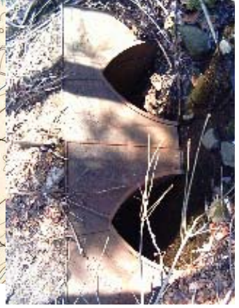
"Munnsville Plow Culvert" - Bridge #402
