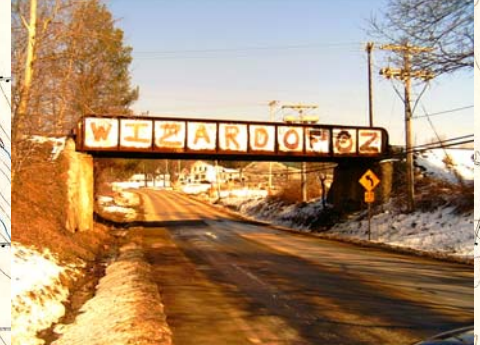
Bridge # 440 on Bypass
