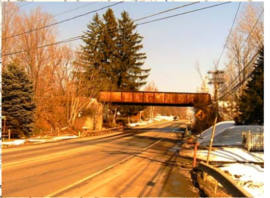
Bridge # 439.5 on Bypass
