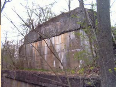
Bridge #358 Over Oneida Creek
