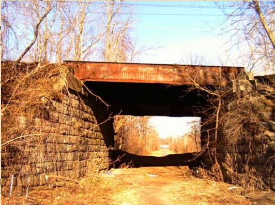
Bridge #357 NYC Overpass of O&W
