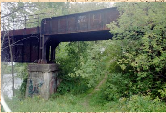
Oneida Castle West Shore Overpass at O&W Station
