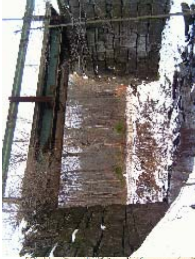
Bridge #395 Over Frederick Creek
