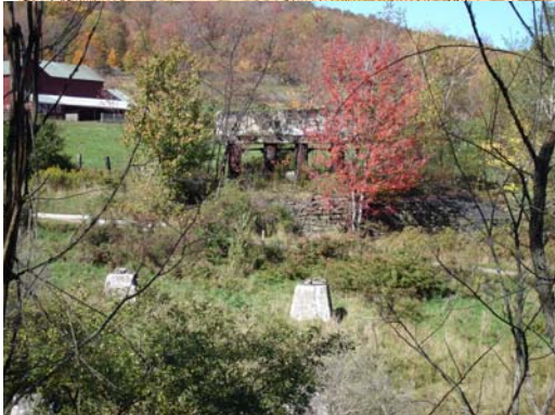
Trestle Supports for Bridge #210
