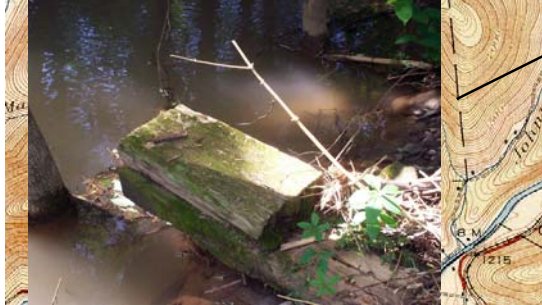
Bridge #179 Support Ties
