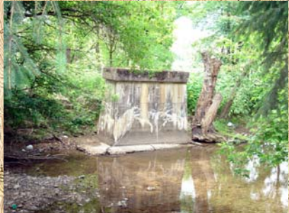
Delhi Branch Bridge #1
