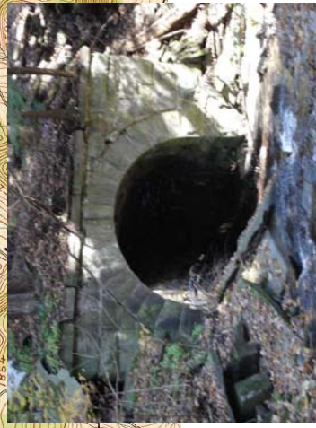
Stone Arch Bridge #228
