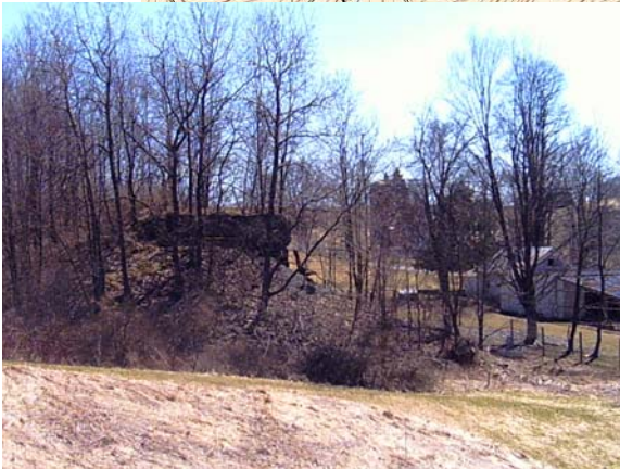
South Abutment Bridge #274
