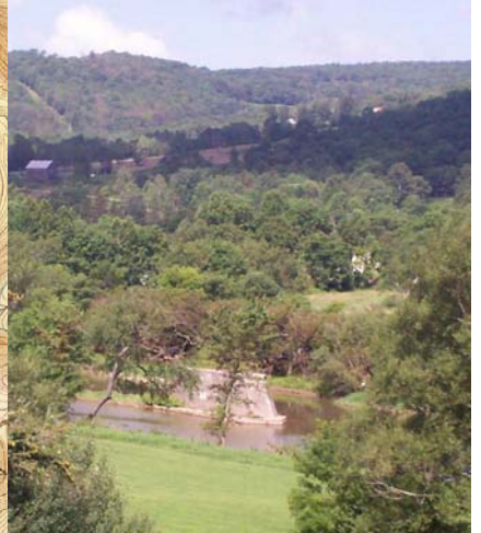
Bridge #182 Over West Branch of Delaware
