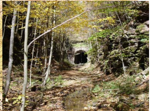
Northfield Tunnel South Portal
